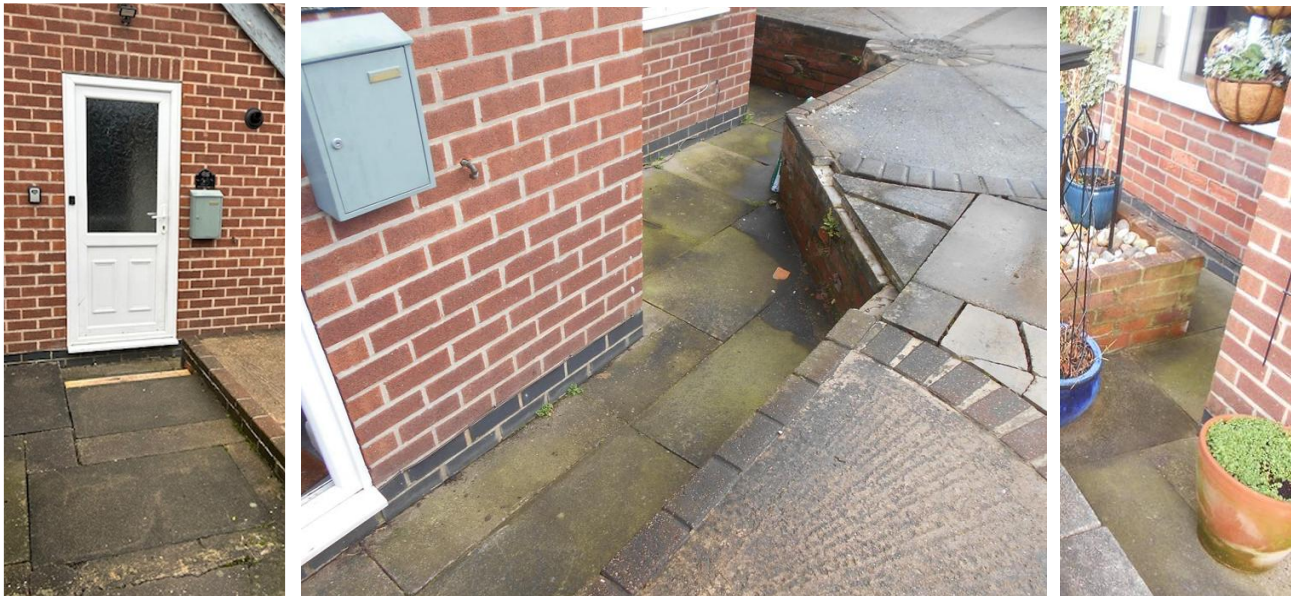
Changes in levels adjacent to the front door
