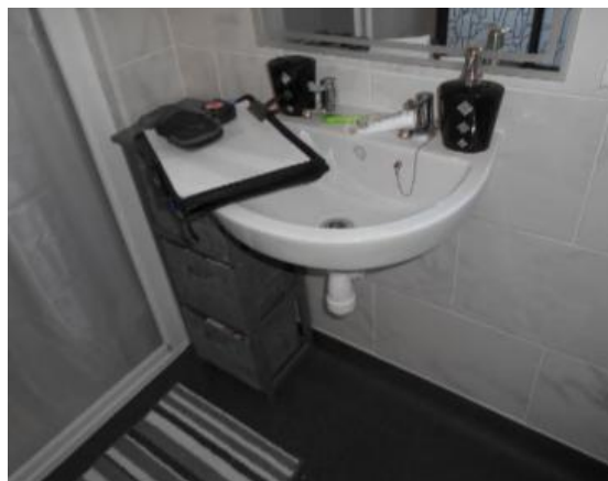
New wall hung WHB (no pedestal) with lever taps
