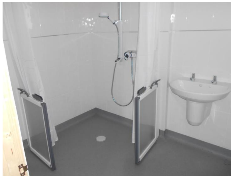
New level access shower area with anti-scald shower, ½ height carer screens, rail, curtain, semi pedestal WHB, slip resistant flooring with coved upstands and fully tiled walls.
