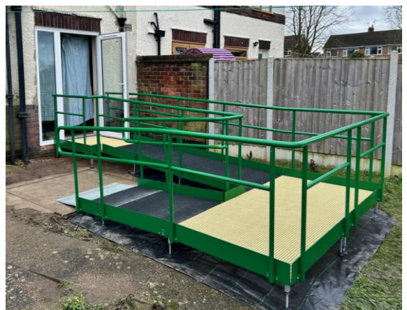
New level threshold back door and ramping
