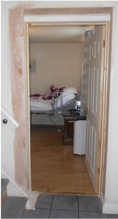
Widened door to GF Bedroom
